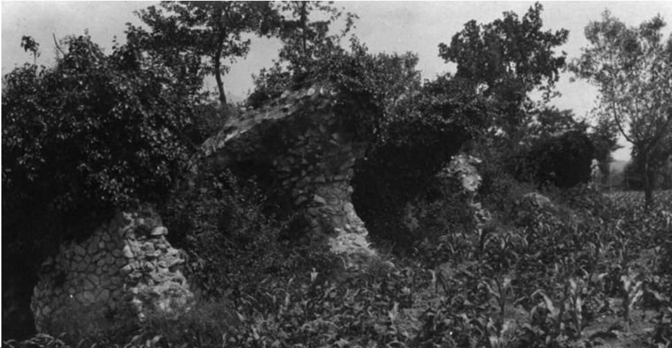
3_Marion Elizabeth Blake, Telesia. Remains of amphitheatre in concrete and opus incertum on road between Venafro and Benevento (Telesia, Italy) , s.d. (Blake Collection, AAR-PA, n. 23).
